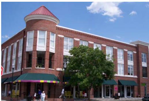
Figure 38 Source: Hall Consulting, Inc.
